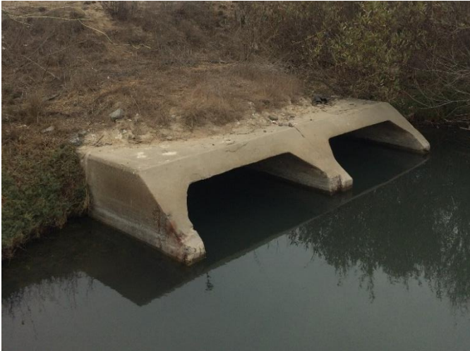
Reach 3 dual concrete culverts
