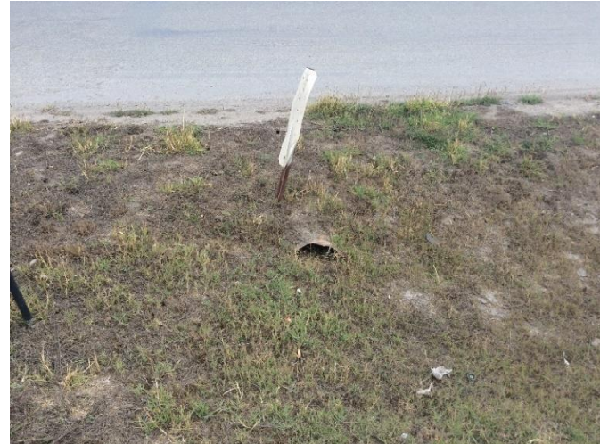
Reach 4 culvert (note structure is filled in)
